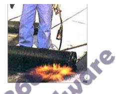
**AquaShield**<sup>®</sup> is normally used in protected roofing and waterproofing applications in a single layer system and is also recommended as base layer in multilayer system in various applications, including damp-proofing.
